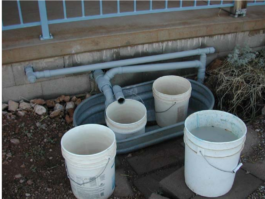
Figure 1. Graywater System in Arizona Where Graywater is Collected in Buckets and Manually Applied to Plant Root Zones.
