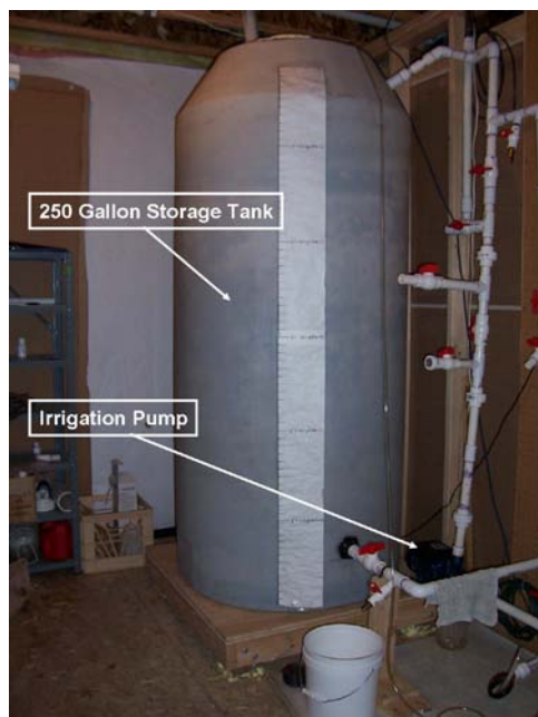
Figure 3. Graywater Storage Tank and Supply to Outdoor Irrigation in Colorado.
