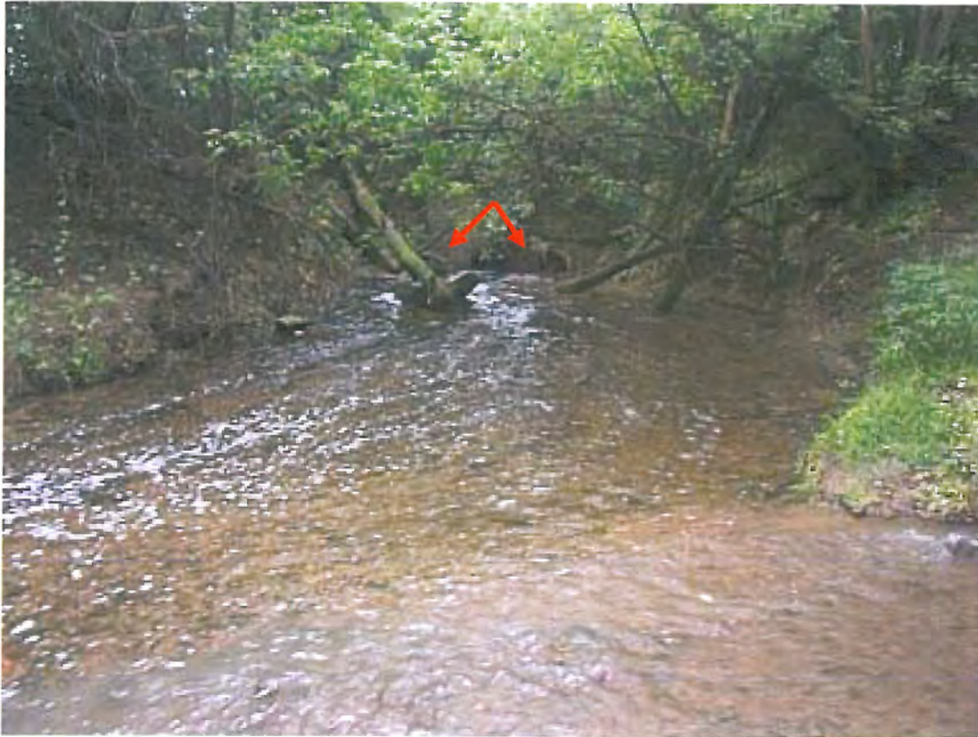
The outfall (red arrows) is located at the head of a 40 foot long drainage into Lytle Creek. The stream bottom consists of gravel and cobbles with areas of silty sand deposition.
