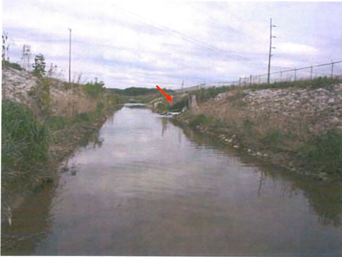
The shoreline around the outfall (indicated by the red arrow) has been stabilized with cobbles.
