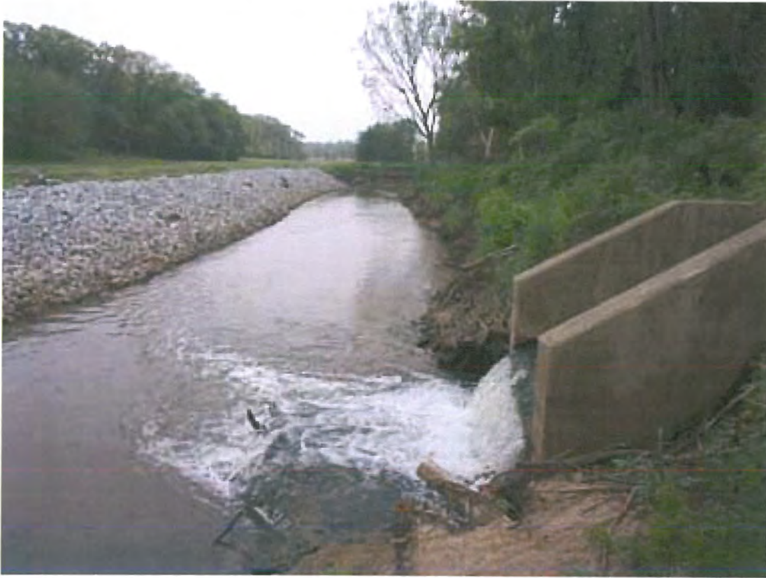
The shoreline near the outfall was cleared of debris and the banks were stabilized with cobbles last year.
