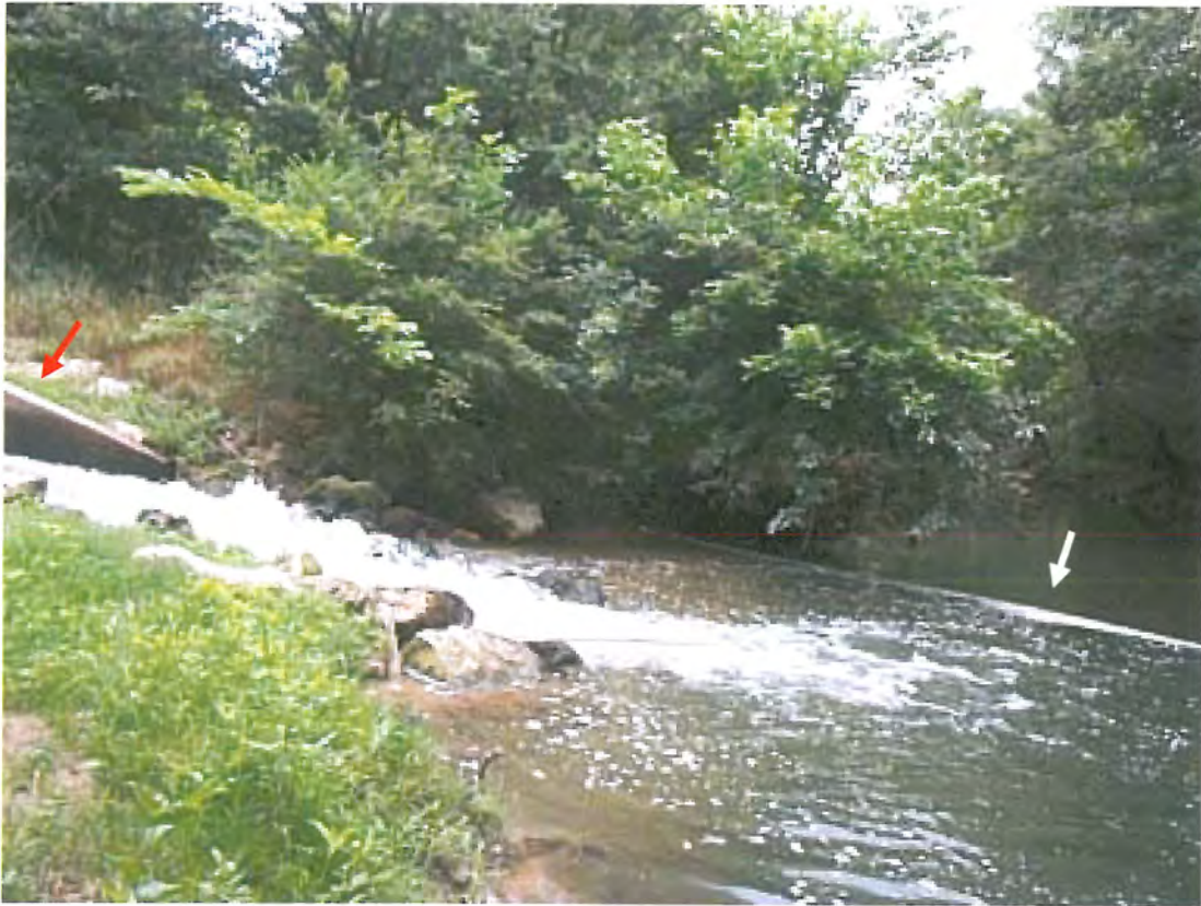
Effluent from the outfall (red arrow) enters a partially impounded portion of the stream that is approximately 3 to 4 feet deep. The white arrow indicates a floating pipe which acts as a barrier for windblown foam.
