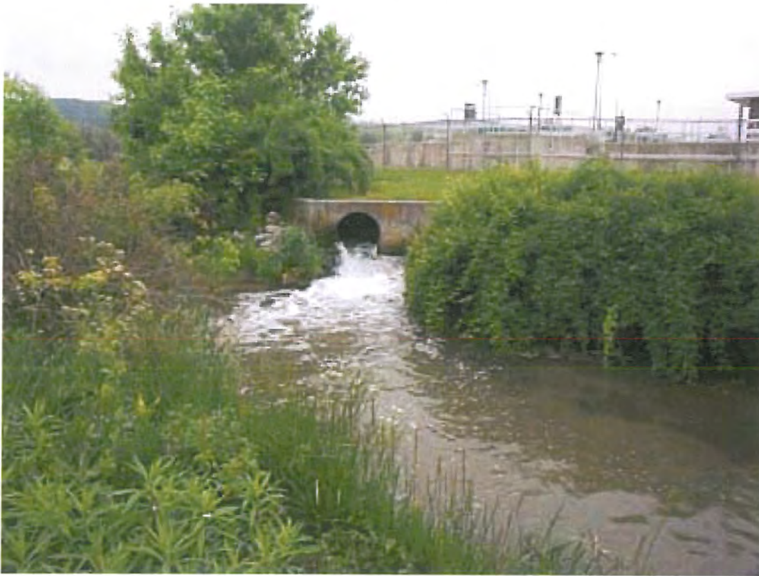
The outfall provides a significant portion of the flow into Little Pipe Creek
