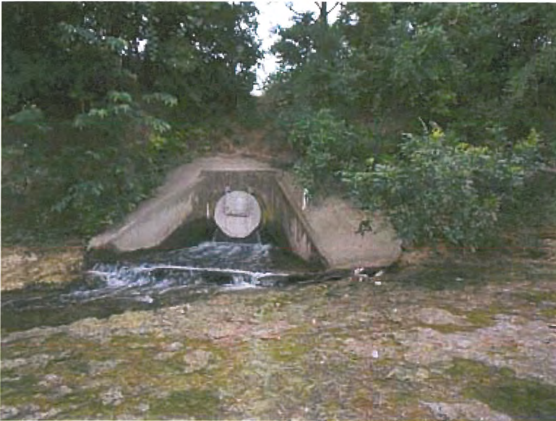
The stream bottom around the outfall is primarily limestone bedrock.
